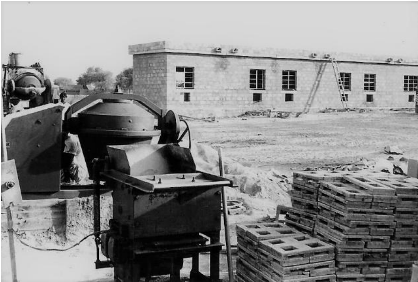
Figure 22 Block making machine. Main concrete mixer and accommodation block in background
