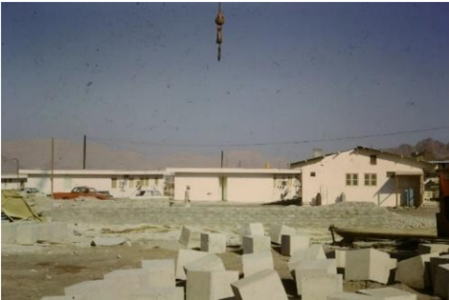
Figure 14 Tarmac compound at Ruwi
