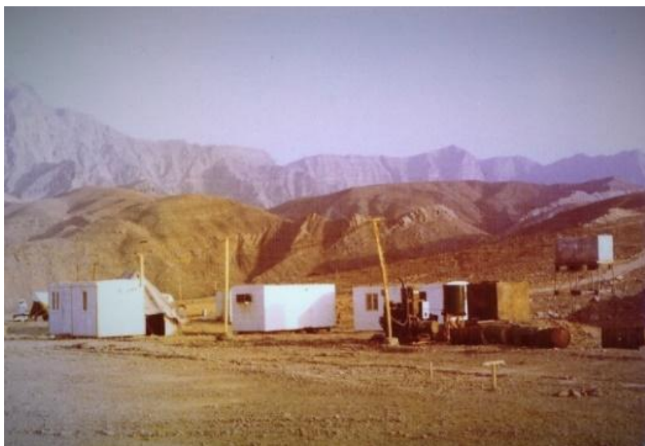
Figure 27 Bukha site set up - day 2
