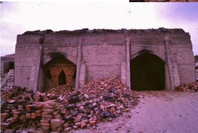
Figure 85a-b Brick kiln. The entrance is walled up and the stacked bricks are fired. It is a slow process.
