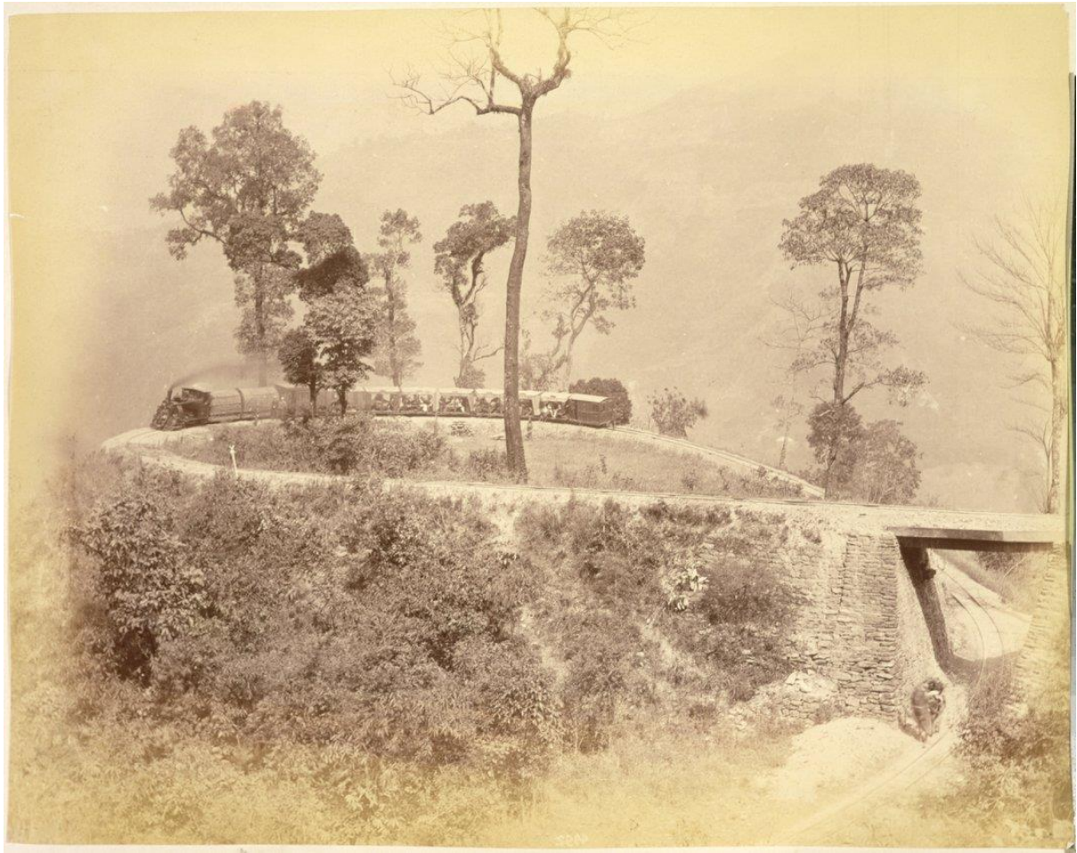
"Agony Point," north of Tingharia, is one of three railway loops along the route of the Darjeeling Himalayan Railway. British Empire and Commonwealth Museum/Bridgeman Images
