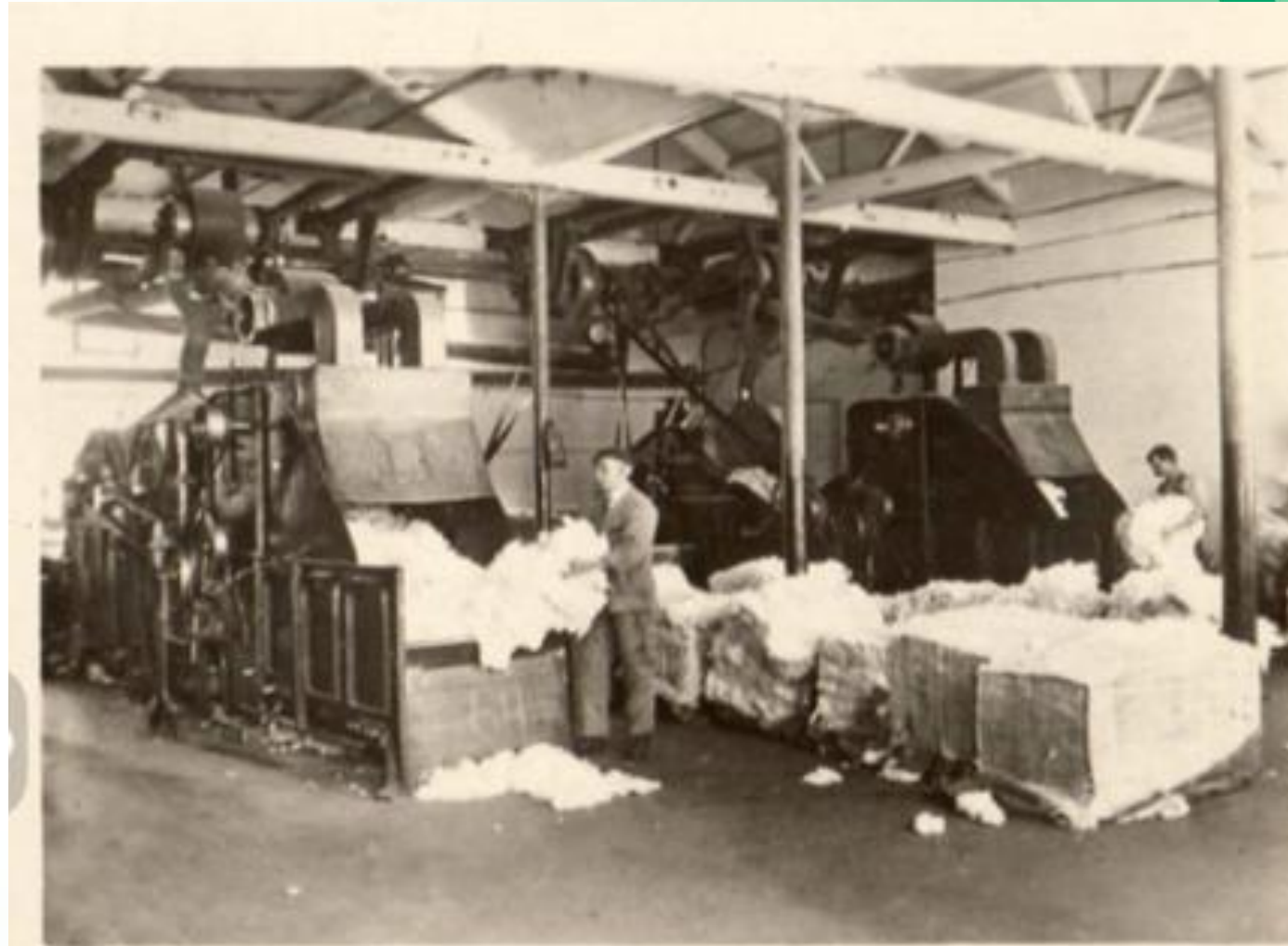
THE MIXING ROOM 11
