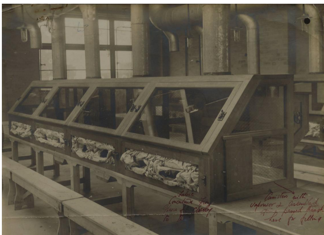
Top. Fig 6. View of White Lund filling shed. The tables on the right are for the canisters after being filled and awaiting completion. Note the overhead sprinklers. All photos The National Archives (TNA) WO 142/116 CWO 114.
